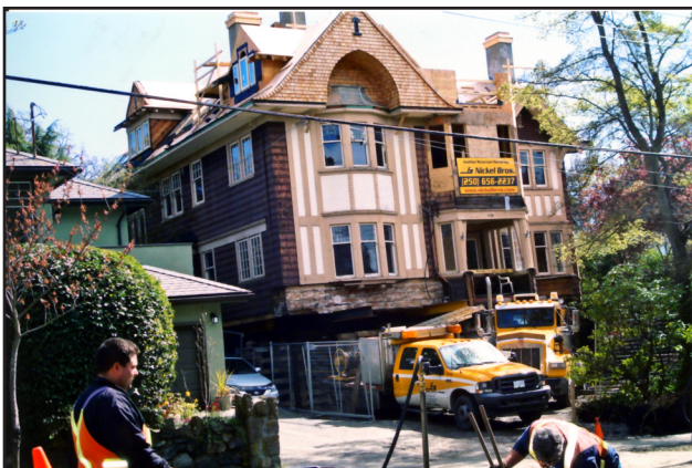
House lifted for new foundation. Steven Chin photo.
