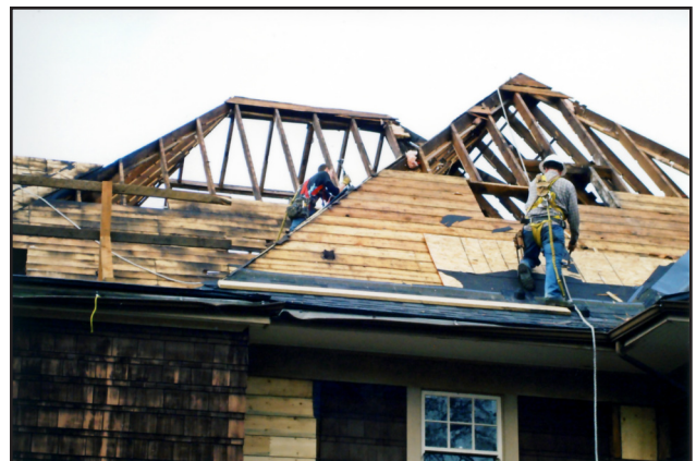
Fire damage, reframing. Photos courtesy Steven Chin.
